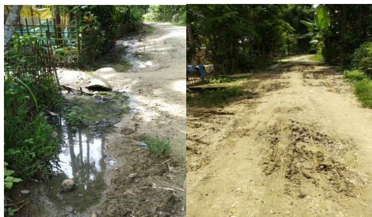
Open drainage system and poor link road (Above)
