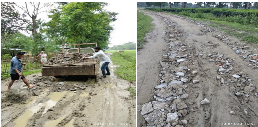
Pre and Post construction images of the road
