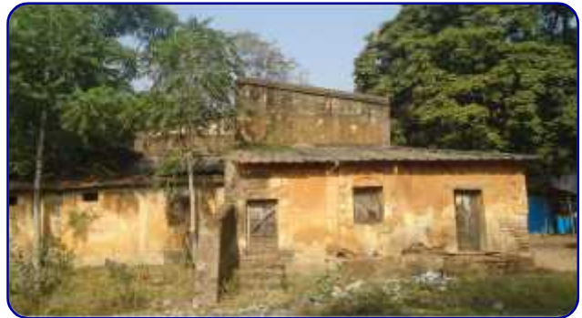
A view of Sahityarathee Bezbaroa's House in Sambalpur. Dibrugarh University organised Bezbaroa's 150th Birth Centenary in Sambalpur with a view that this creates a platform for due preservation of this heritage house.
